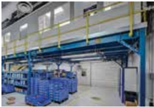
Lab on Pre-Engineered Mezzanine
