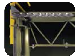
Truss Girder & Bar Joist
