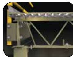
Beam & Bar Joist
